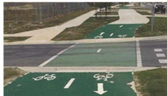
Note: Example of a separated bike way that has been designed and constructed on Timbertop Boulevard, Officer.
