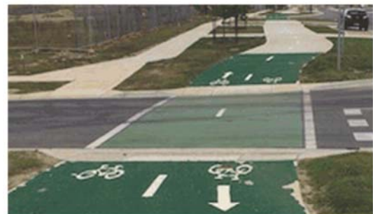
Note: Example of a separated bike way that has been designed and constructed on Timbertop Boulevard, Officer.
