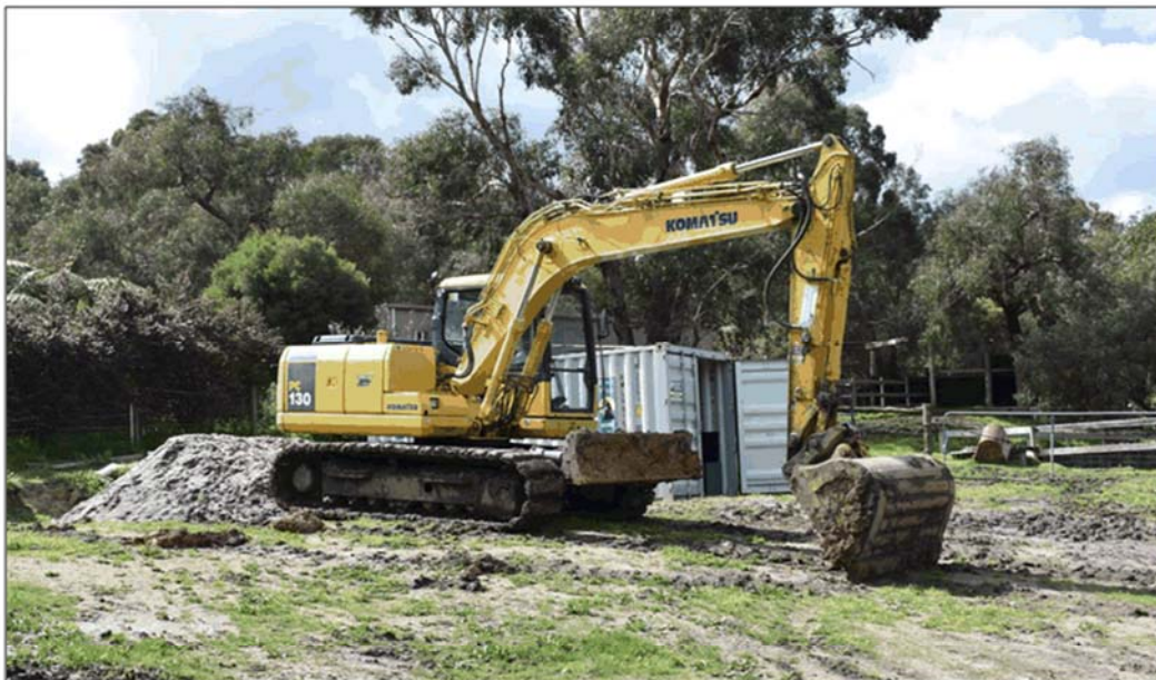
Photo 2: Owners large excavator located on the subject land.
