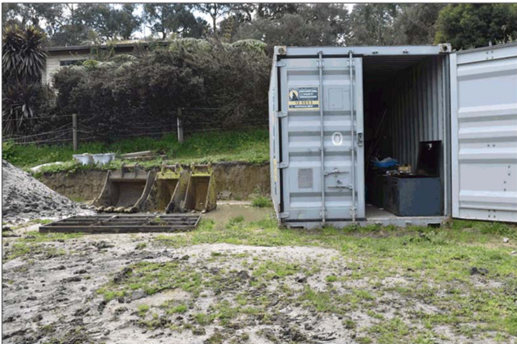
Photo 4: Various attachments used by the excavators.
