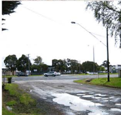
GLISMANN ROAD & PRINCES HIGHWAY EXISTING INTERSECTION
