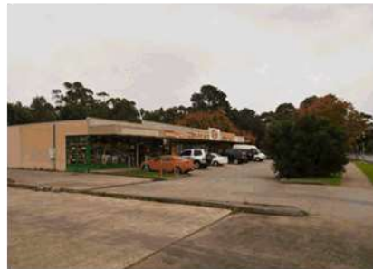
EXISTING SHOPS ALONG PRINCES HIGHWAY
