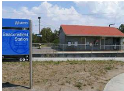
BEACONSFIELD RAILWAY STATION
