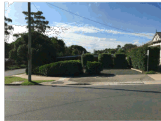
P6 2 SALISBURY ROAD EXISTING SINGLE STOREY DWELLING BRICK VENEER - PRESSED REDS SHEET ROOF - SILVER
