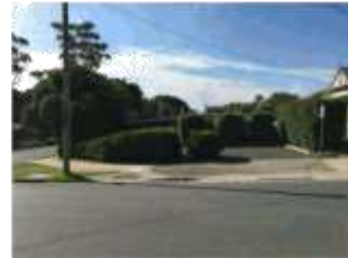
P6 3 SALISBURY ROAD EXISTING SINGLE STOREY DWELLING BRICK VENEER - PRESSED BRICK SHEET ROOF - SILVER
