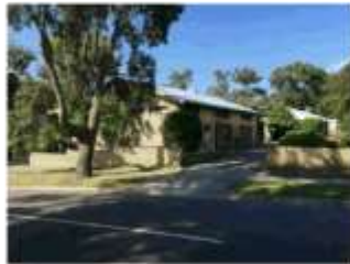
P1 34-36 BEACONSFIELD-EMERALD ROAD EXISTING SINGLE STOREY DWELLING & ASSOCIATED SHED TIMBER WEATHERBOARD - NATURAL (SHED) SHEET ROOF - SILVER (SHED)
