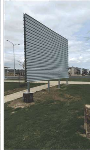
Looking towards Princes Hwy.
